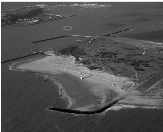
Fig. 3 Station “Kabeltonne” on Helgoland Roads (54°11.3'N, 07°54.0'E) between the main island of Helgoland (in the background) and the “Düne” (photograph: P. Mangelsdorf)
