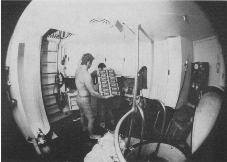
Fig. 4: Two aquanauts in the Tektite wet room prepare for an excursion. The relatively large space permitted up to four divers to suit up simultaneously. Other room features include a shower (left side), ladder to other compartments, scuba tank charging station (right side wall), and the entry trunk
