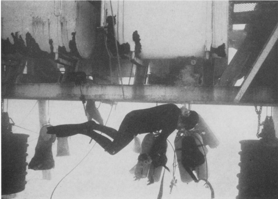
Fig. 6: Holding his breath, a diver swims down from the Edalhab entry trunk and dons his scuba system hanging beneath the habitat. Surface support divers returned empty cylinders to the surface for refilling
